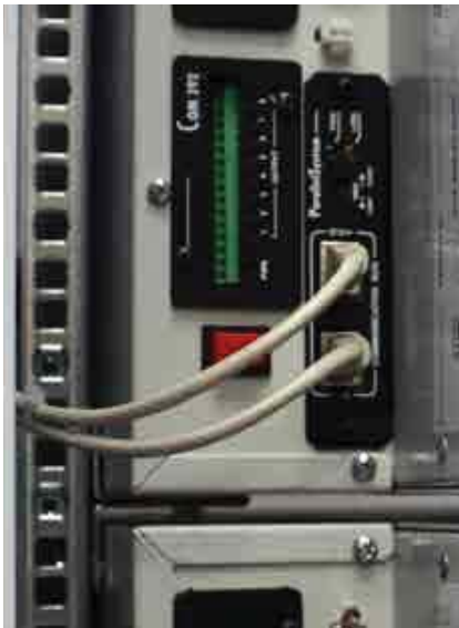
Parallel configuration and programmable relay contacts board.
